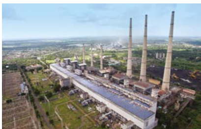
Kolaghat Thermal Power Station
