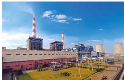
Sagardighi Thermal Power Plant
