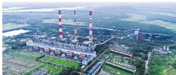
Bakreshwar Thermal Power Plant
