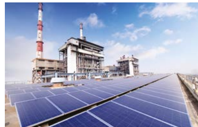
Santalidih Thermal Power Station
